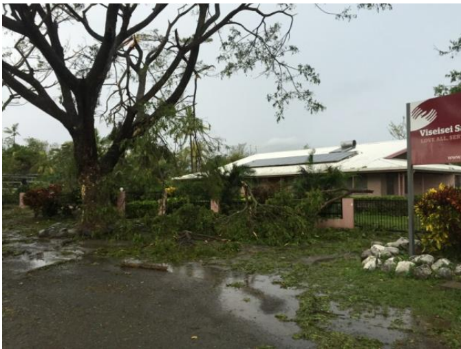
Front of the Health Centre
